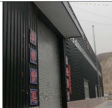
封闭厂房+15m 排气筒
